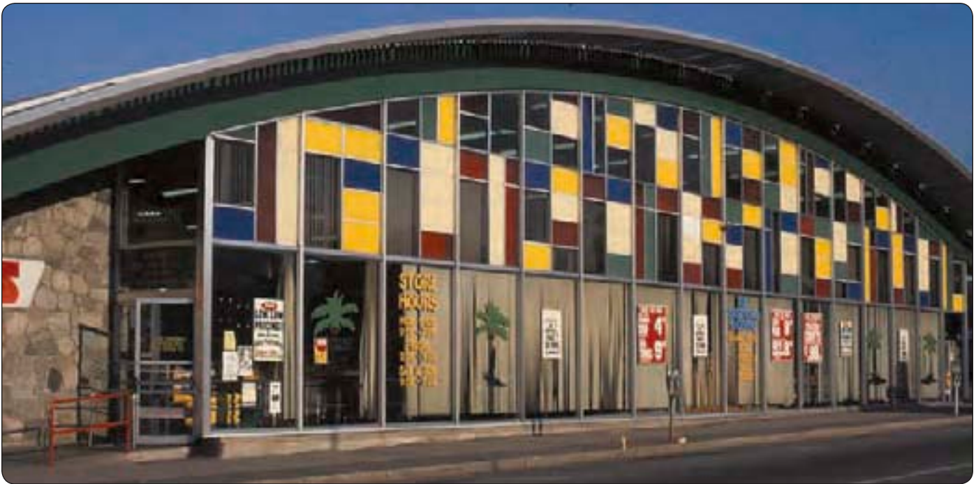
Super Valu on Martin Street, since removed, featured a classic arch lam beam construction. D. Cox photo.
