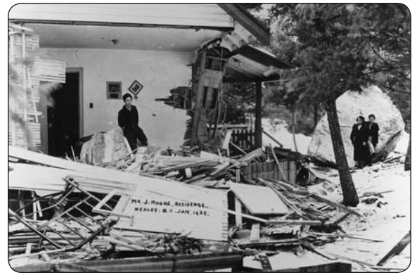
The Jack Moore residence in Hedley after the rock slide from Stemwinder Mountain January 24, 1919. The Vancouver Sun, January 25, stated, "...photo shows what remains of the bedroom of two of the four children of Mr. and Mrs. Jack Moore. The children were asleep in the room when the slide started and ran from the room just before a huge boulder crashed into it." Dave Innis photo collection.
