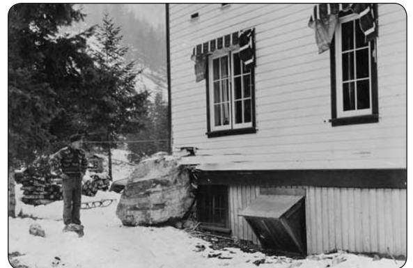
The Tremaine home with a huge rock that stopped beside their house. The opening on the side of the house is a coal chute. Coal and sawdust were used to heat homes.
